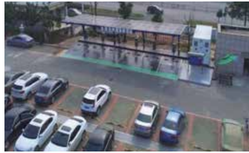
Solar & ESS & Charging station
