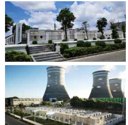
Utility ESS · Transmission & Distribution side
